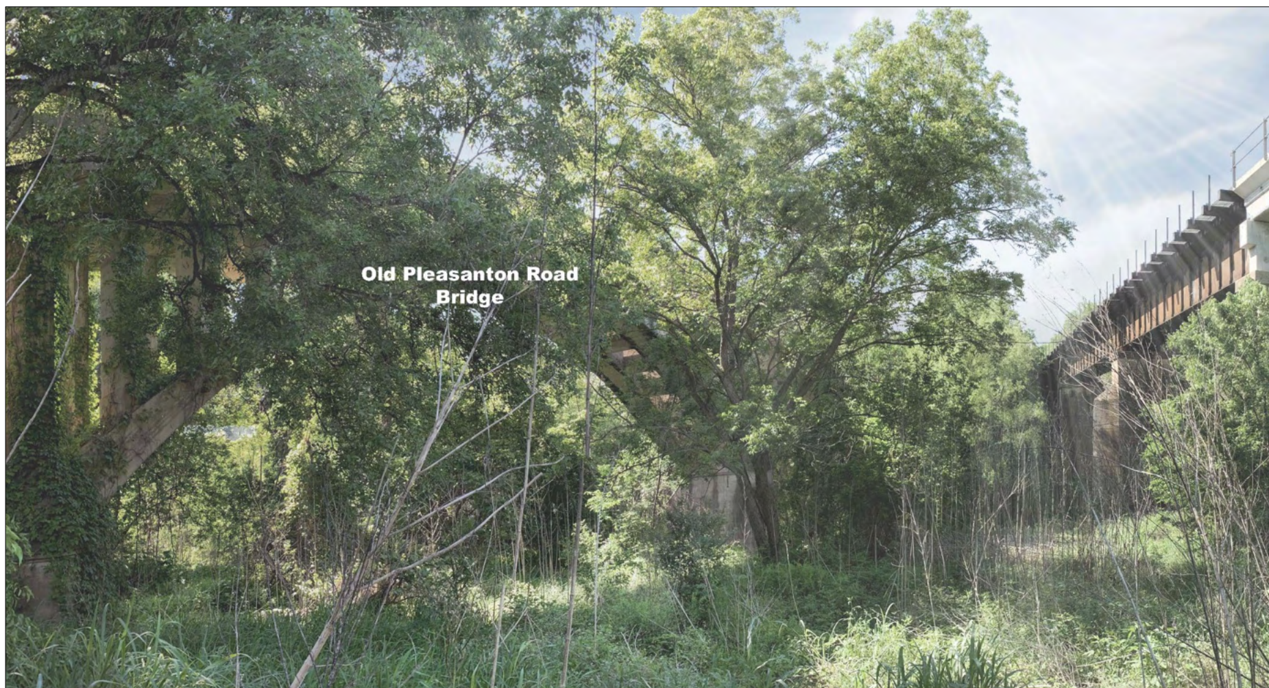
Figure 14: Focus Area #3 Transformative Project – Old Pleasanton Road Bridge (Existing)
